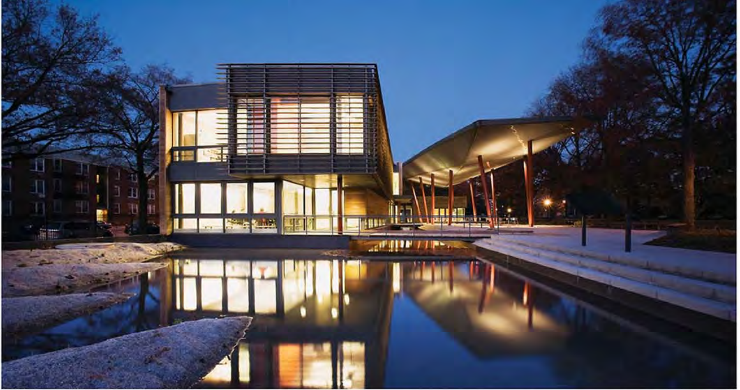
Queens Botanical Garden Visitor and Administration Center was the first new public building in New York to achieve LEED Platinum certification from the Washington, D.C.-based U.S. Green Building Council. PHOTO COURTESY OF JEFF GOLDBERG/ESTO
